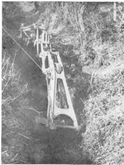
40. The Ditching Grab entering the ditch
