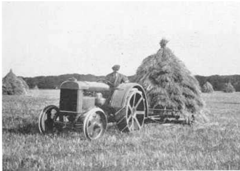
26. A special sweep brings a complete Tripod 'hut' to the thresher
