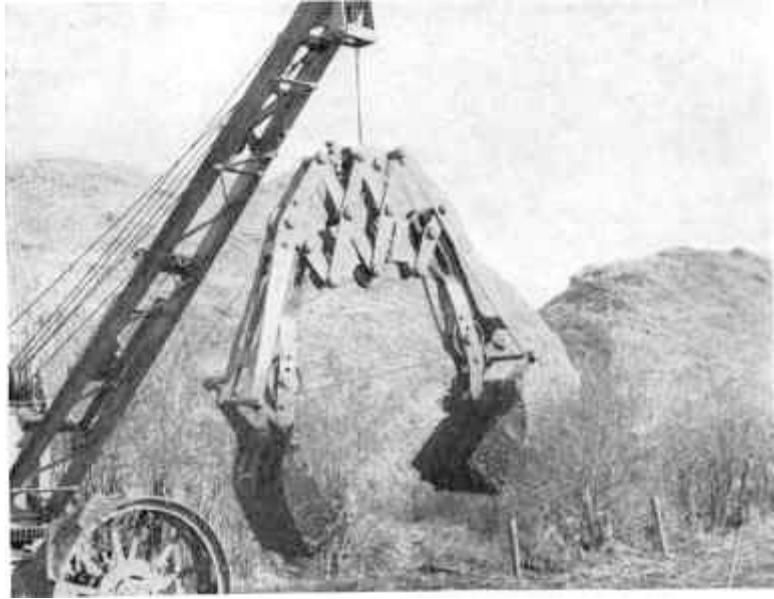
39. The Ditching Grab half extended
