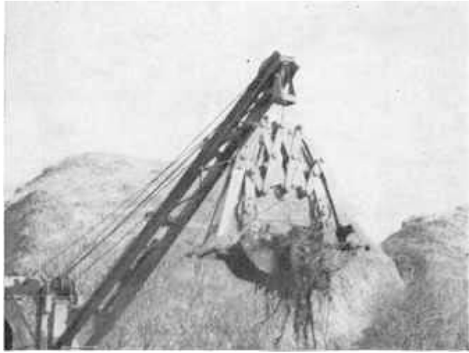
41. The Ditching Grab loaded
