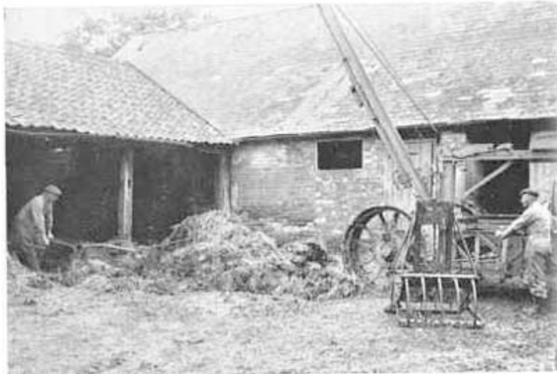
14. Rapier Muck Shifter, removing muck from underneath a low building
