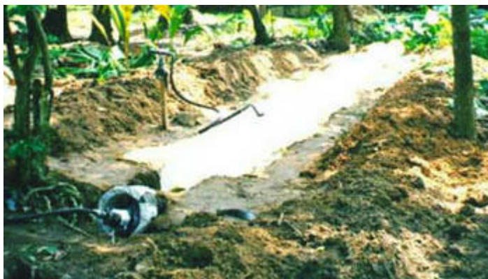
Figure 10. Photo of a biogas plant, filled with exhaust and water.
