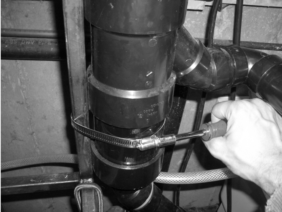
Photo #18 Adjusting exhaust manifold height.
