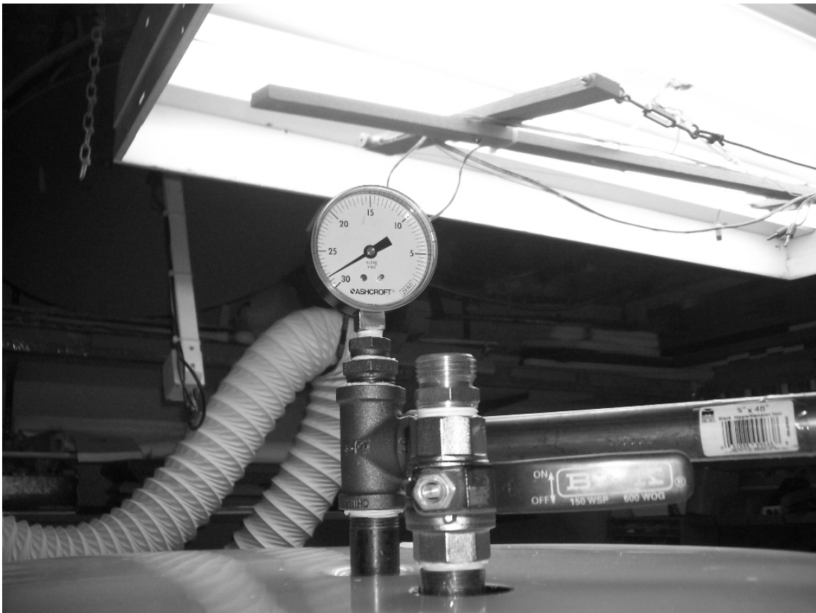
Photo #17 Checking system ultimate vacuum.
