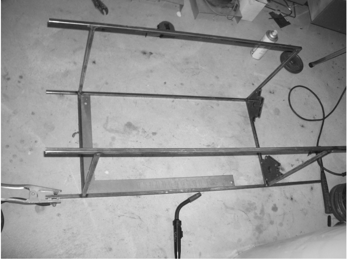
Photo #11 Frame fit up.
