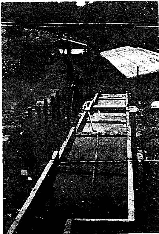
Illustration 2-5: Sludge conditioning canals with overflow dams.
