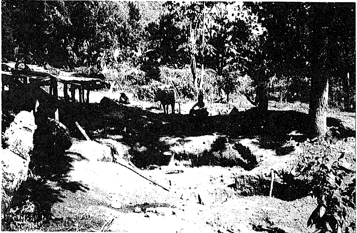
Photo 11: A nearly finished fixed-dome plant in combination with cattle shelter (Source: OEKOTOP, BEP Tanzania)
